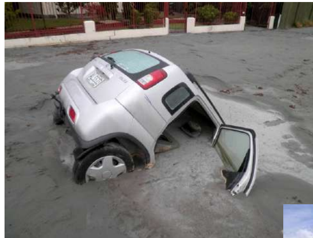
Liquefaction in Christchurch: CEISMIC Digital Archive (Mark Lincoln)
